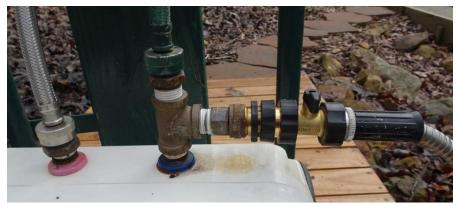
3326X8 Brass CA360 Fitting, Nipple, 1/2" NPT Male, Close," one "Anderson Metals Brass Garden Hose Fitting, Swivel, 3/4" Female Hose x 1/2" Female Pipe," and the male member from the garden hose quick disconnect set.
