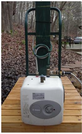
Use the channel-lock or slip-joint pliers to tighten all water hose connections.
